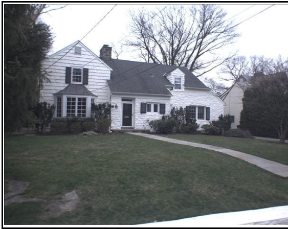
4 Locust Ridge Rd 553289 1-9-301
