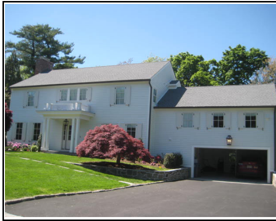
2 Well House Ln 553289 3-40-608
